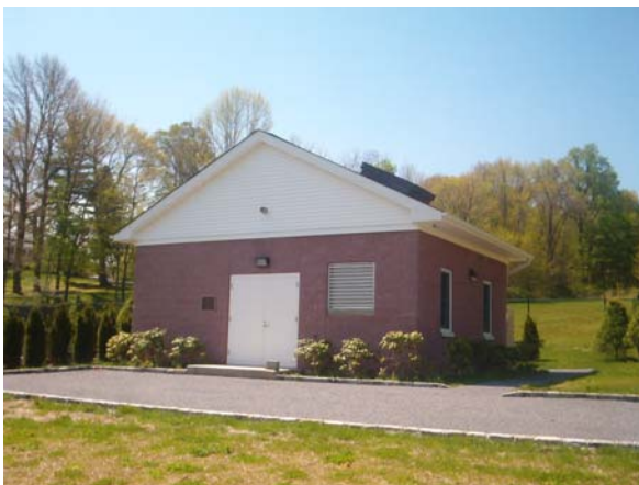
New Well House No. 2-2 – Shutter Lane
