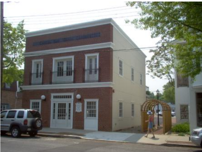
Completed Renovations of District Office
